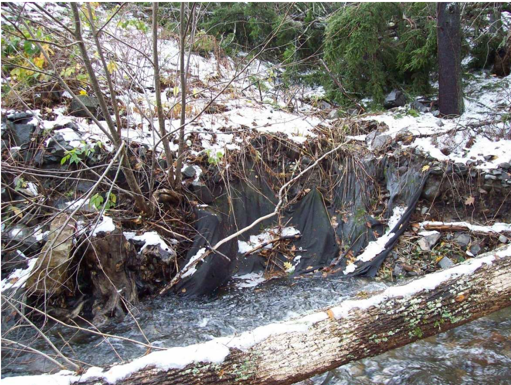
Upstream view erosion of river right channel bank (November 5, 2014)
