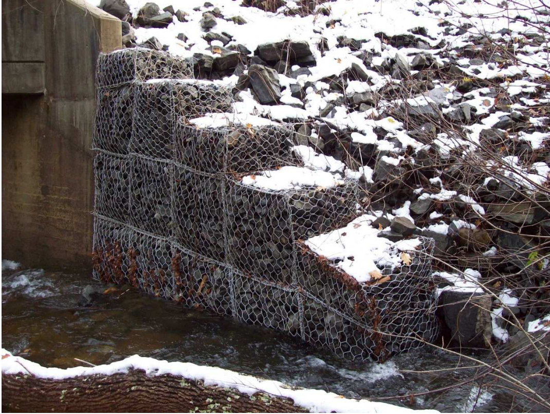
Upstream gabions that are leaning in towards the stream (November 5, 2014)
