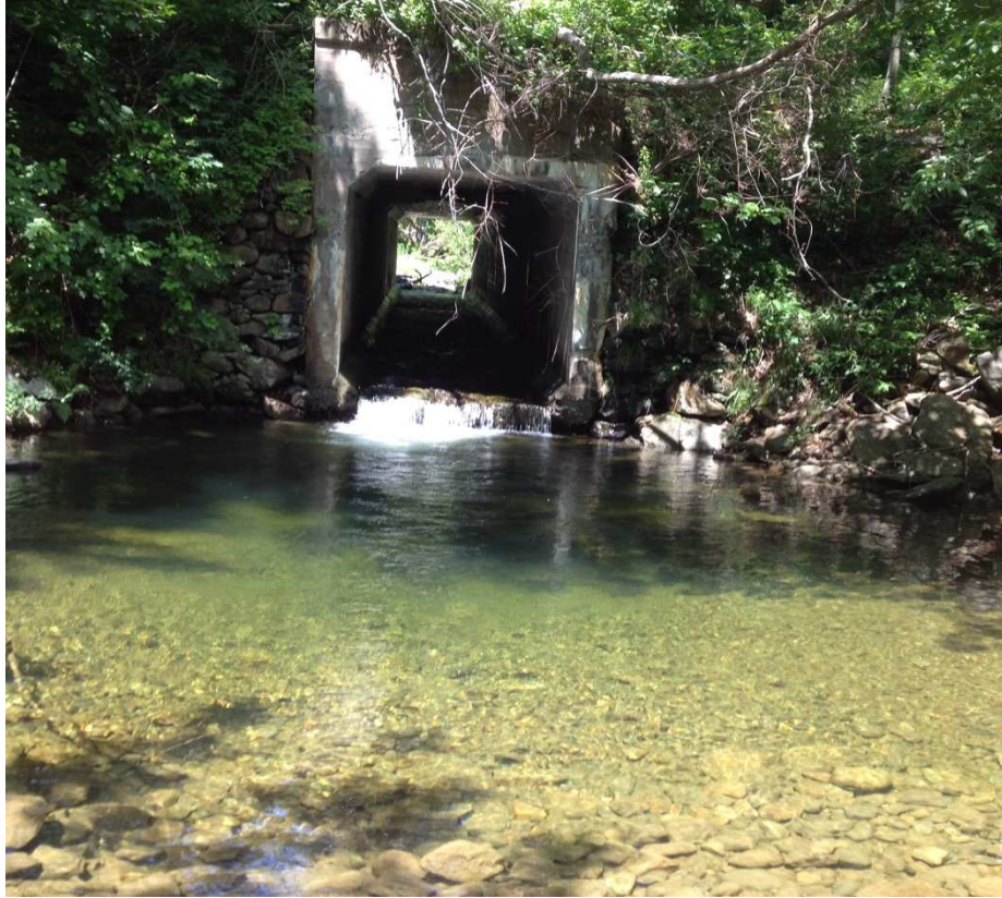
Scour hole looking from downstream (June 30, 2015)
